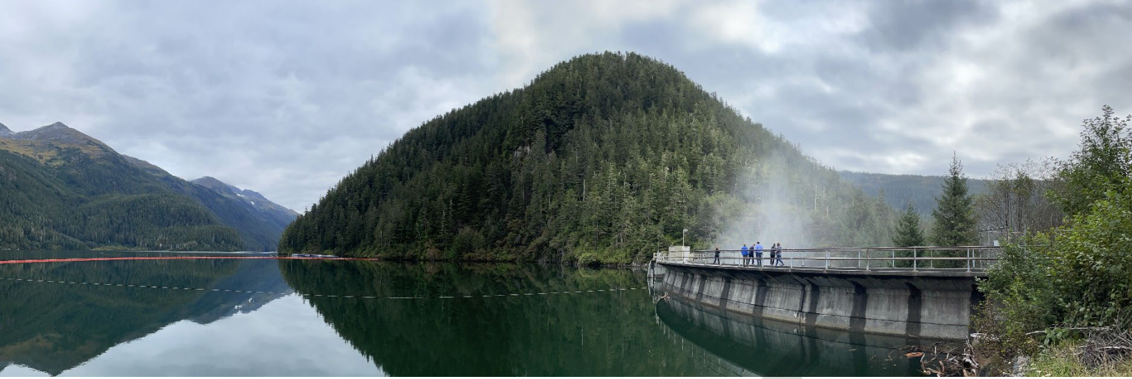
View of the reservoir behind the Green Lake Hydroelectric Project
